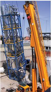
POLARIS proposed that Liranco (help) set up a solventseparating system consisting of two distillation columns and an extraction column, all on skids, but working together as an integrated unit.
