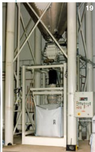
Waste material silo which fills FIBCs for underground storage
