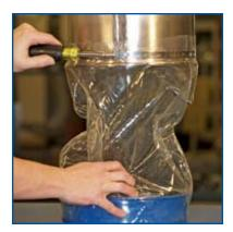
1. Securely band clamp the ROTEX PolyClear Sleeve to the upper pipe and let the sleeve hang down. The material is designed to be stretched over the pipe for a snug fit. If a little more room is needed, diameters can be easily increased by briefly using a hot-air gun when installing.
